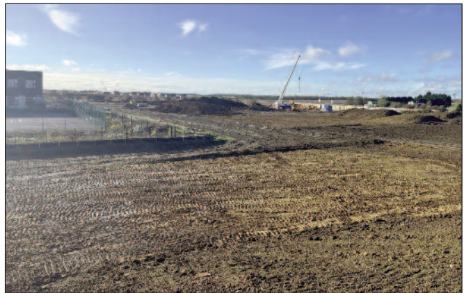
EARTH-MOVING: A huge amount needs shifting to create playing field surfaces.
